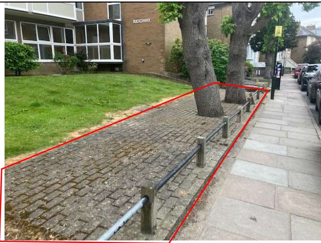
Paving to be retained.
