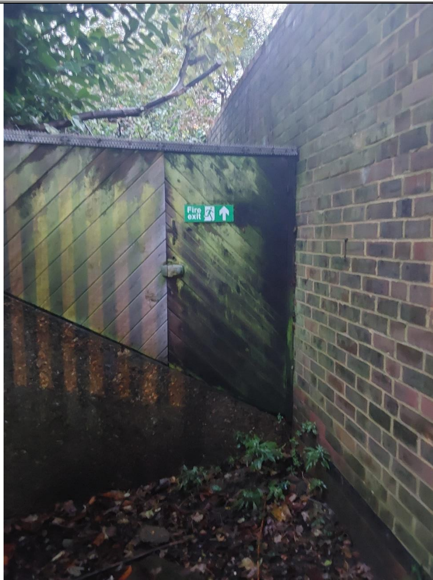
Rear exit from garage into next door garden.
